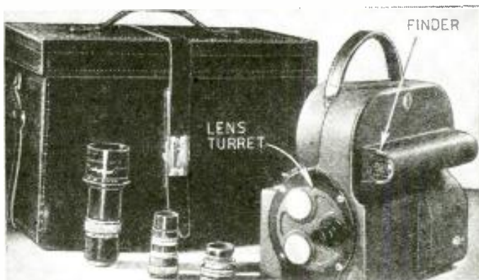
The sound camera with its carrying case and lenses.
