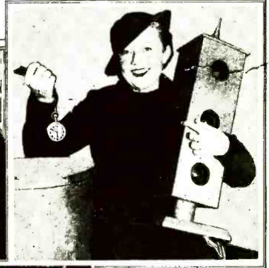
↑ This young lady is holding a new device—a stop-go signal for public speakers. The light turns yellow, then red at the end of the allotted broadcasting time.
