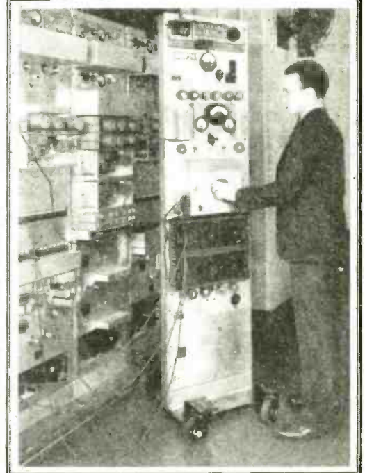
→ Another transmitter development appears at the right. It is a portable transmission measuring set, containing an oscillator with an equalized output which is flat from 50 to 9,500 cycles. Measurements can be made between losses of 80 db. and gains of 75 db. to an accuracy of 0.1 db. Western Electric photo.
